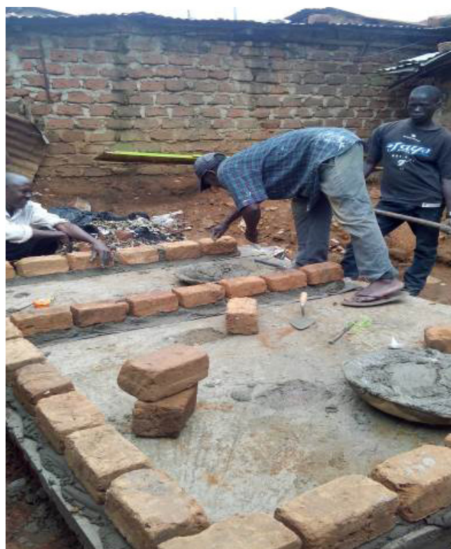
PHOTO 28: BUILDING PIT LATRINES ACCORDING TO KCCA MINIMUM STANDARDS
