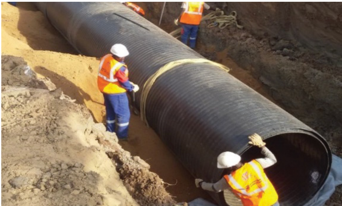
PHOTO 16: SEWER BACKBONE NETWORK BEING LAID IN KAMPALA, NWSC, 2018
